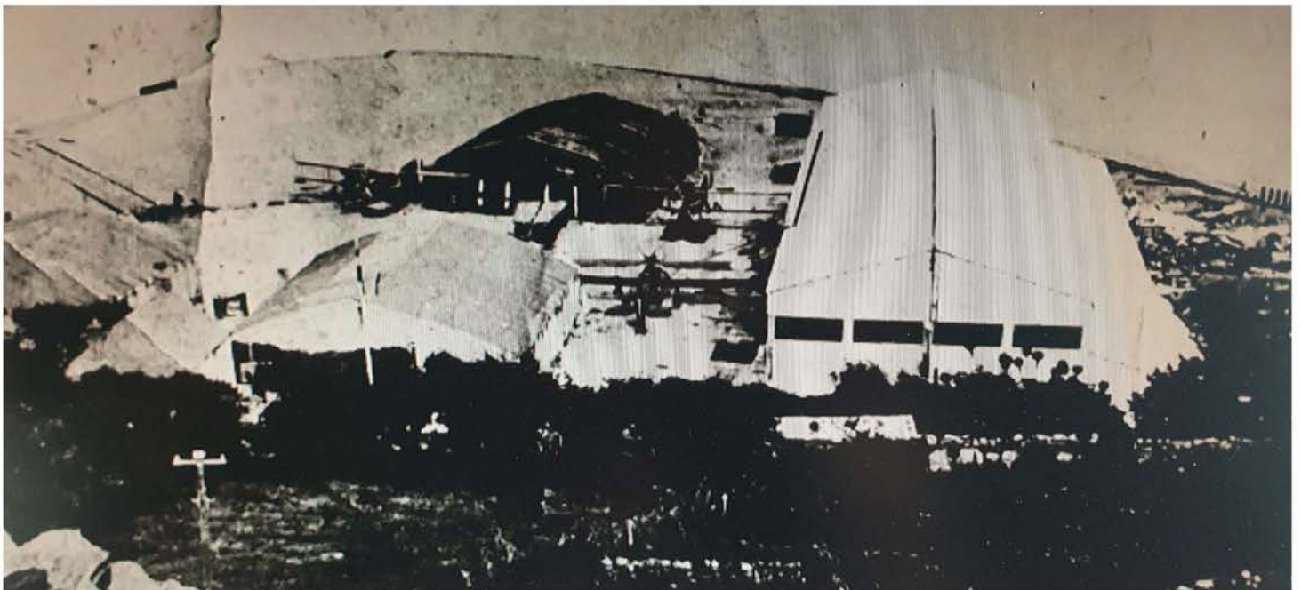
A view of the base from the west (poor quality photo but it gives you an idea of how cramped everything was.)
