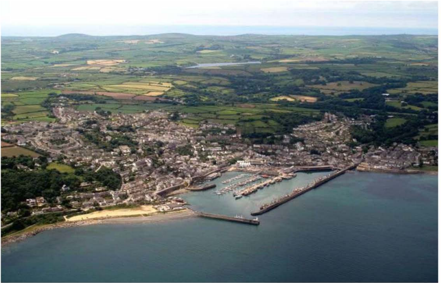
A more recent aerial view of the site of RNAS Newlyn and it shows how much erosion has taken place over time and the promontory has completely disappeared.
